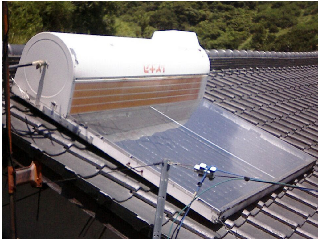
Figure 1. “Taiyounetsu Onsui Ki - Taiyounetsu de Mizu wo Atatamete Kyuutou nado ni Riyou Suru Tame no Souchi (Solar Water Heater -- A Device to use for Hot Water Supply, etc. -- Heating Water Using Solar Heat).” Solar Thermal Heating System. Solar Thermal Heating System. Source: Toto-tarou - Own work, Wikimedia commons. CC BY-SA 3.0 , August 1, 2006. Accessed August 10, 2020. https://commons.wikimedia.org/wiki/File:TaiyonetuOnsuiki.jpg#/media/File:TaiyonetuOnsuiki.jpg
